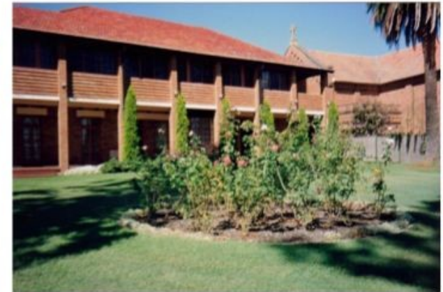
Another view of Monte Pio Motor Inn
